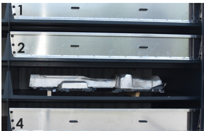
4 floodable compartments for damaged batteries
